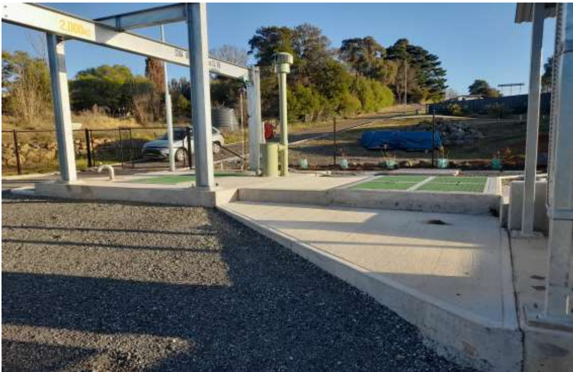
Photo 4.3 Wellington Road SPS (December 2021)
