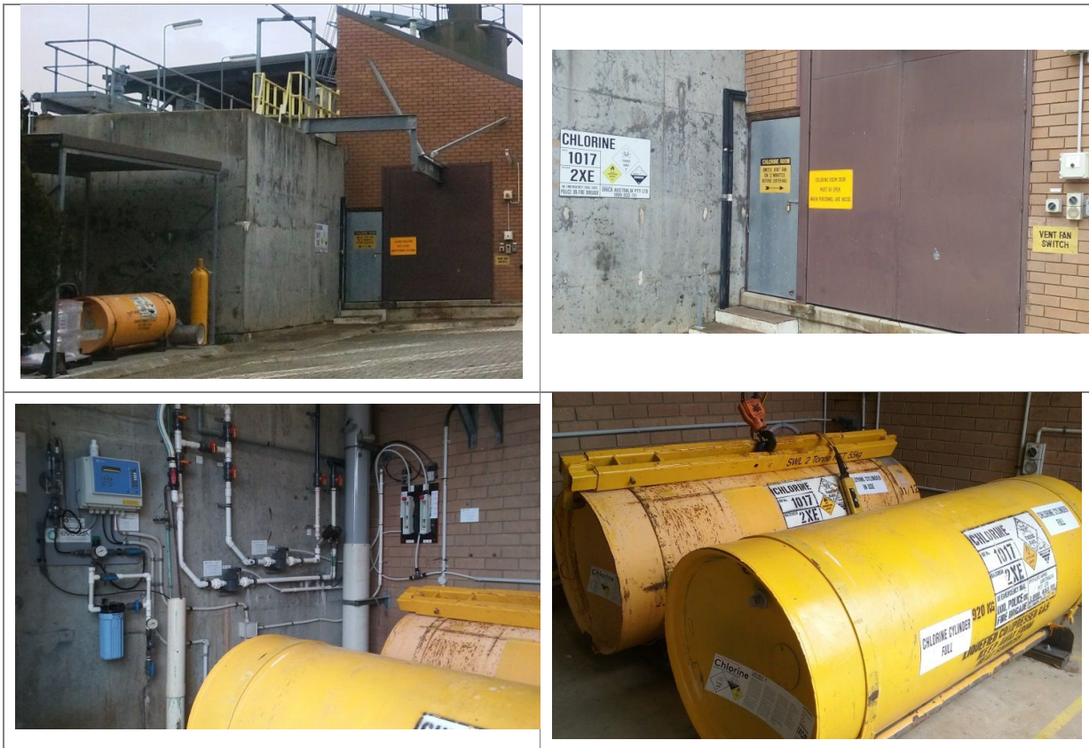
Photo 4.4 Chlorine Gas Storage and Dosing Area
