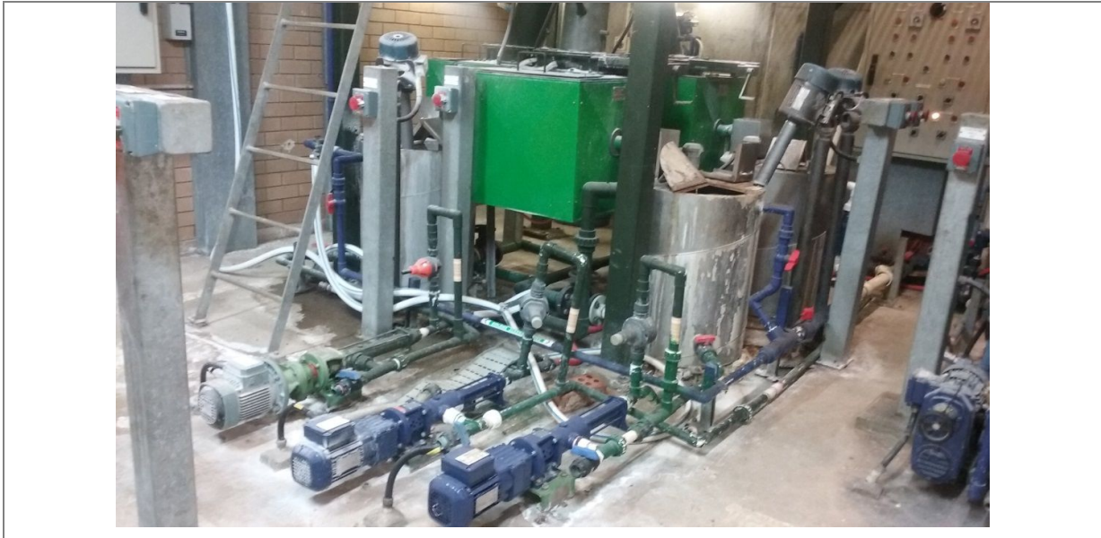
Photo 4.3 Soda Ash Storage and Dosing Area
