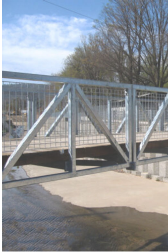
Steel truss pedestrian bridge (image from Landmark)
