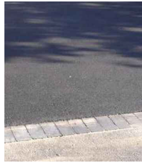
ASPHALT FOOTPATH WITH GREY BRICK TRIM
