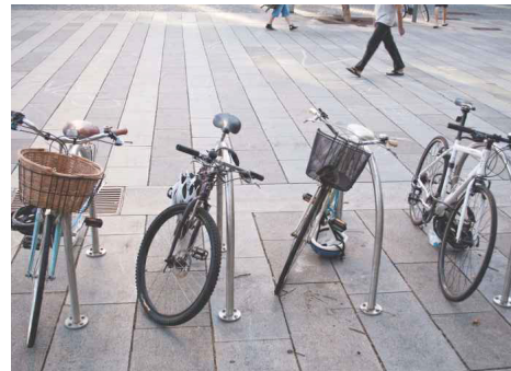
CYCLE RACKS: Street Furniture Australia, Semi-Hoop, galvanized or stainless steel
