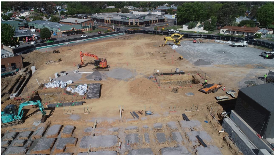
Figure 1 & 2: Library Stage 1 and 2 – Inground Services & Slab Works
