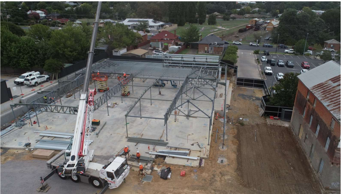
Figure 1 Library Structural Steel installation
