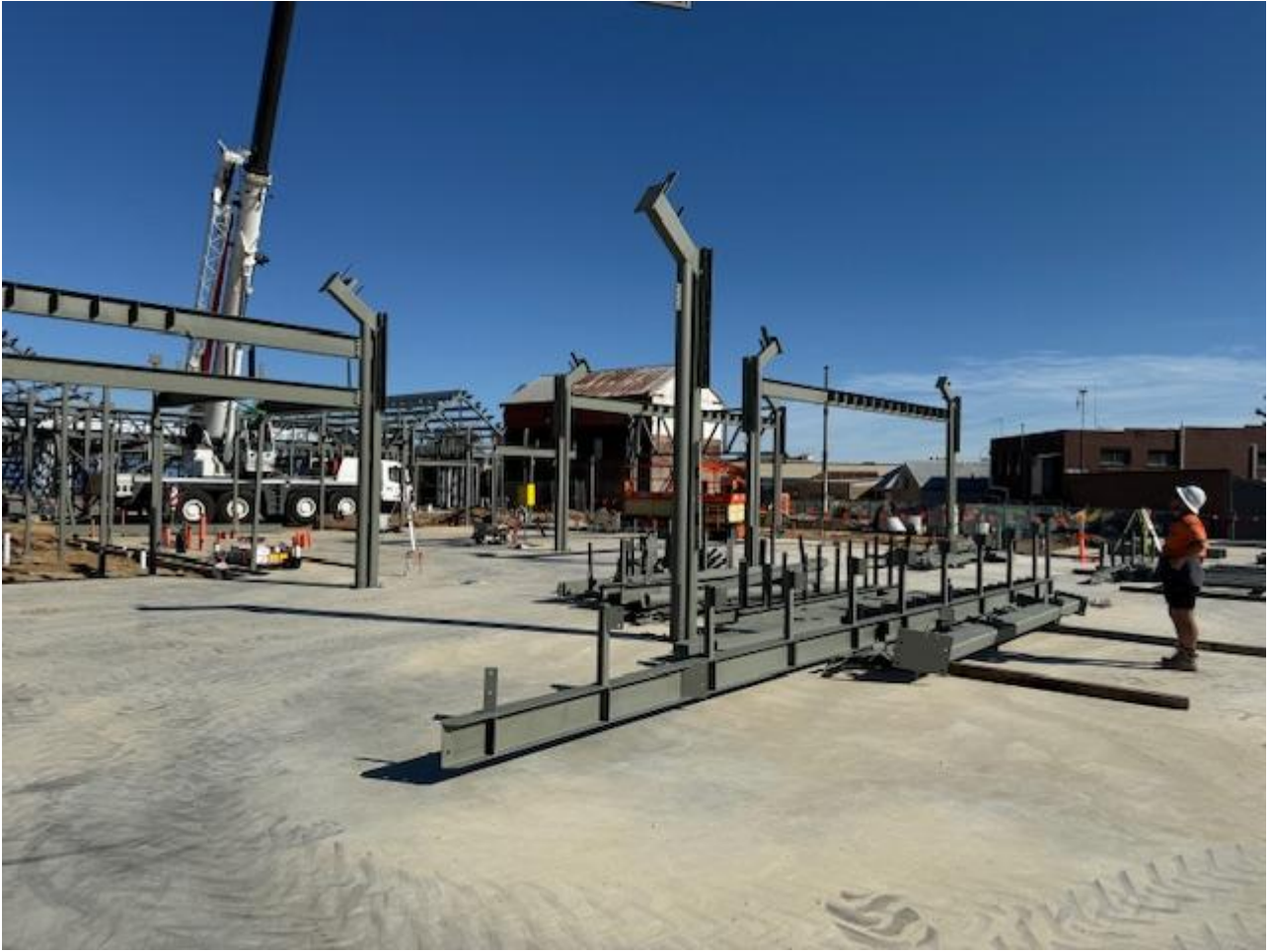
Figure 2 & 3 Admin Structural Steel installation
