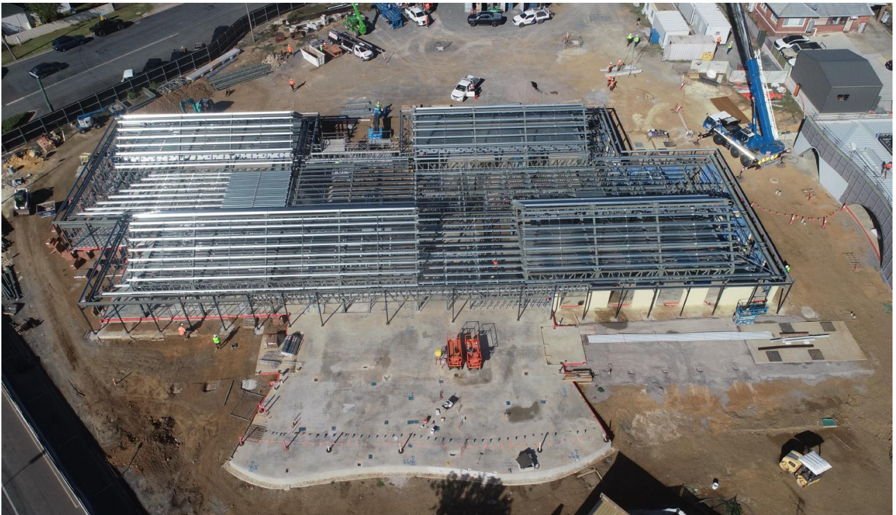
Figure 2 Administration Building Structural Steel Works
