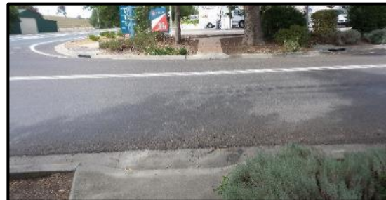
Plate 44 - Kerb Ramps Hercules Street Murrumbateman
