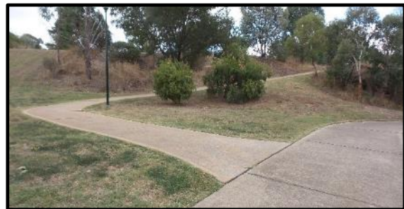
Plate 8 – Dutton Street Link
