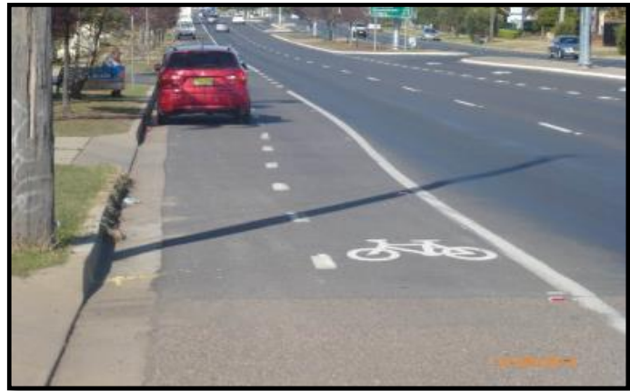
Plate 2 – Typical on-road cycleway
